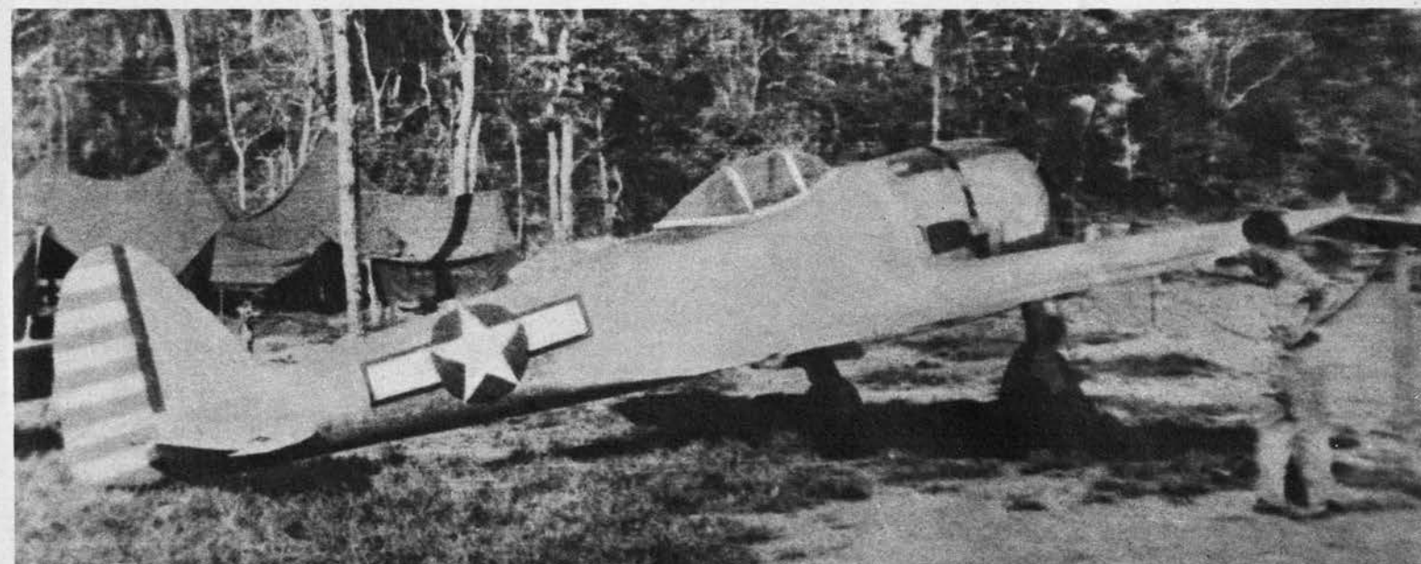
OSCAR 2 Most frequently seen Japanese Army fighter, Oscar has been given new heavier armament, a new engine and a modified wing since it was first introduced. Guns are
